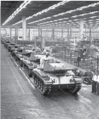
Rolling off the line at the Cadillac Tank plant in Cleveland.
